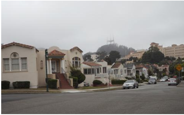
100 and 200 blocks of Vazquez Street in Forest Hill Extension.
