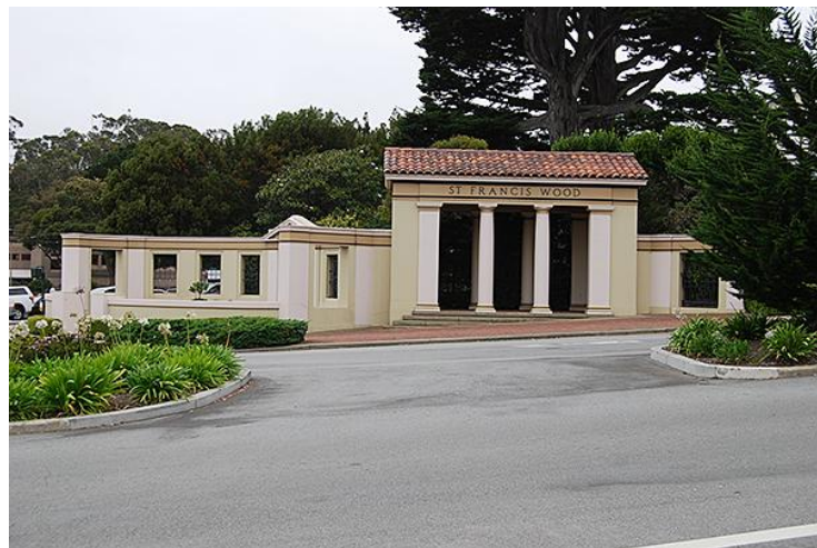
North side of Main Entrance at St. Francis Wood and Junipero Serra Boulevards.
