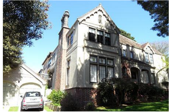
1600 Monterey Boulevard, St. Francis Wood
