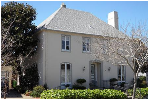
2 Santa Ana Avenue, St. Francis Wood
