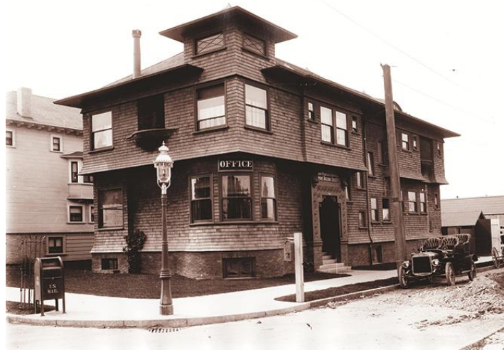
Sales office of the San Francisco and Suburban Home Building Society in Jordan Park. The building is extant as a residence at 101 Jordan Avenue at the corner of Euclid Street. (Western Neighborhoods Project collection)
