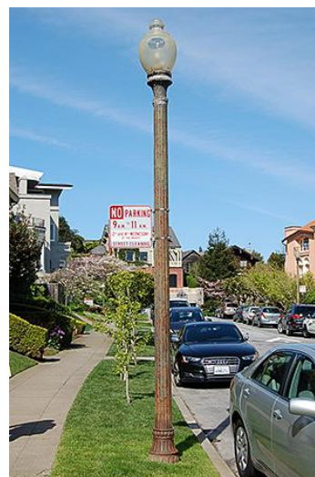
Example of historic streetlight on West Clay Street.
