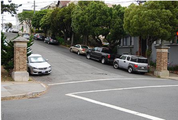
36th Avenue entrance structures.
