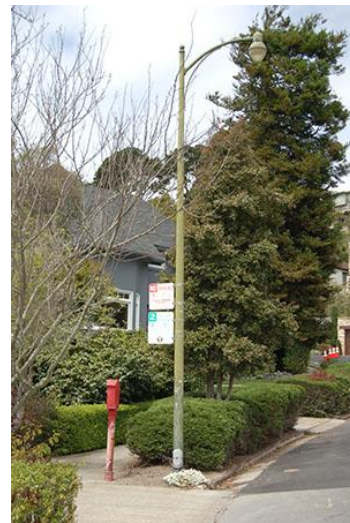
Example of streetlight on Montalvo Avenue. (Note the teardrop globe has often been retrofitted with a cobra light.)
