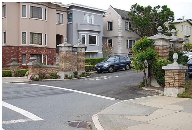
Main Entrance Gate at 37th Avenue and Geary Boulevard.
