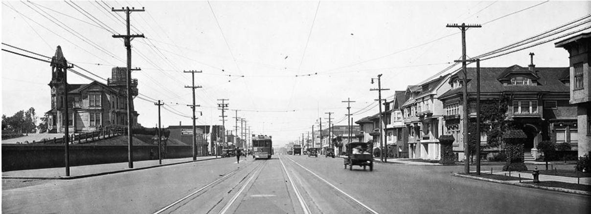
Jordan Park residences and entry pillars on right (not extant), across Geary Street from the Odd Fellows cemetery (not extant) and crematorium, August 1925. (Bancroft Library, University of California, Berkeley)
