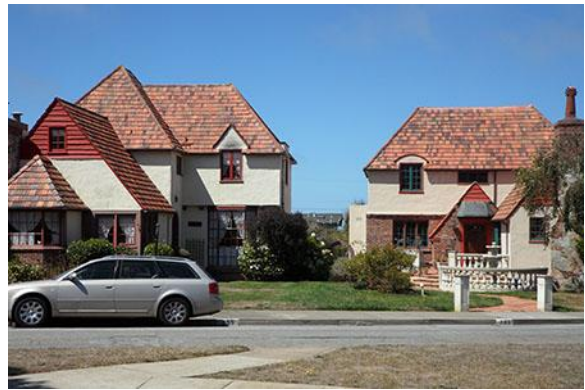
255 and 266 Moncada Way, Ingleside Terraces
