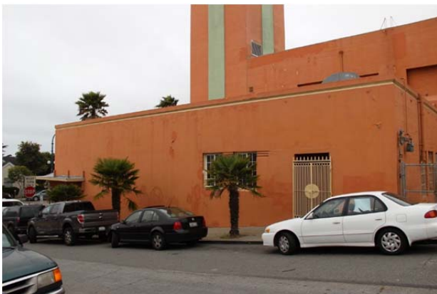
Figure 12. East wall of east retail wing, looking southwest.
