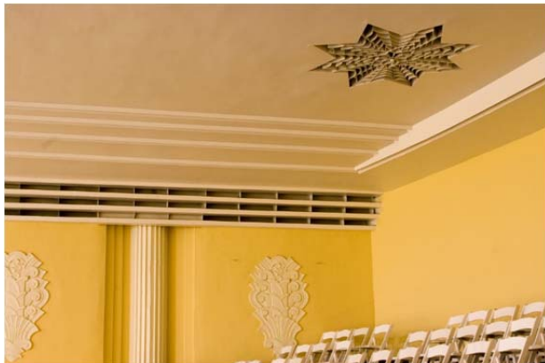
Figure 22. Detail of Auditorium walls and ceiling, looking east
