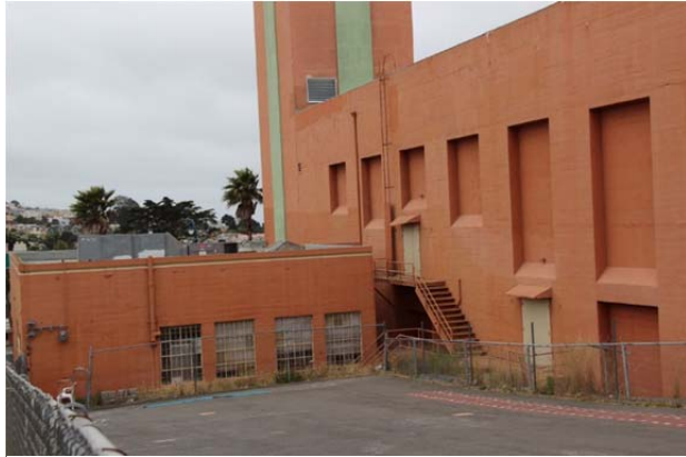
Figure 14. North wall of east retail wing, looking south.
