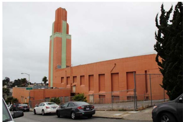
Figure 13. East wall of auditorium, looking southwest.
