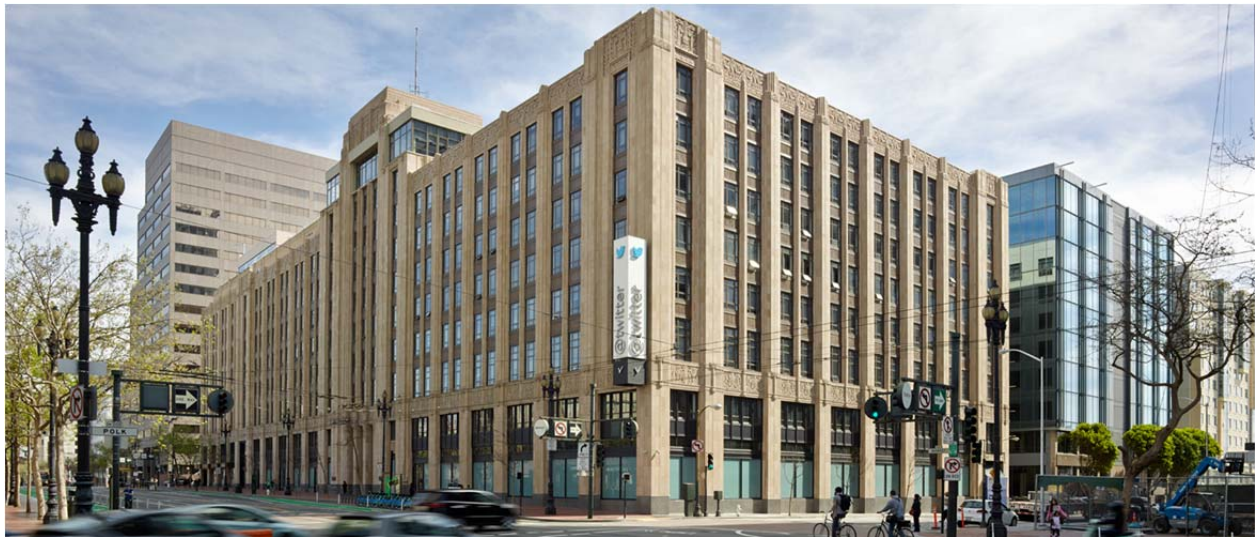
Figure 49. Western Furniture Mart, aka, the "Twitter Building."
