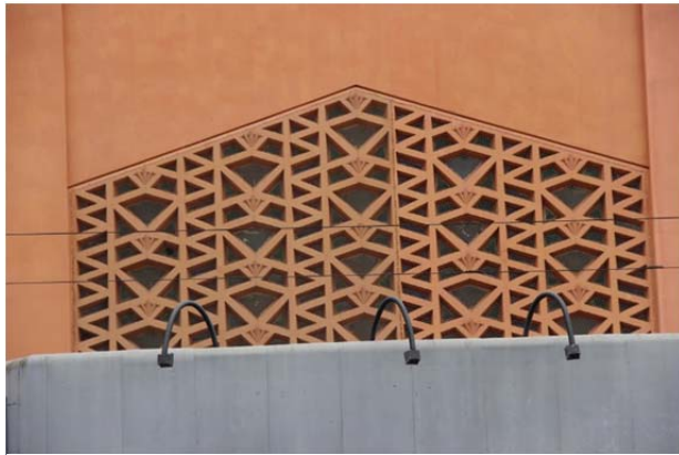
Figure 8. Concrete grille above main entrance.
