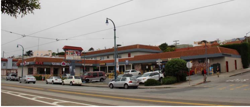
Figure 3. Strip mall on Ocean Avenue west of Lakewood Avenue.
